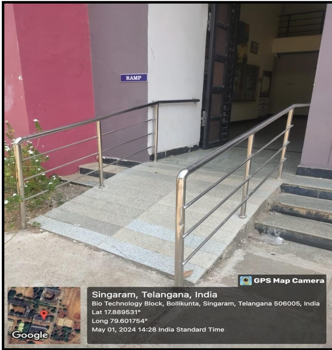
Ramp Provision for Disabled students and Employees
